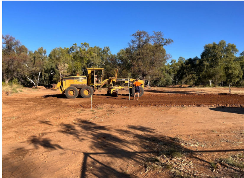
Above: Workers repairing the community access road
