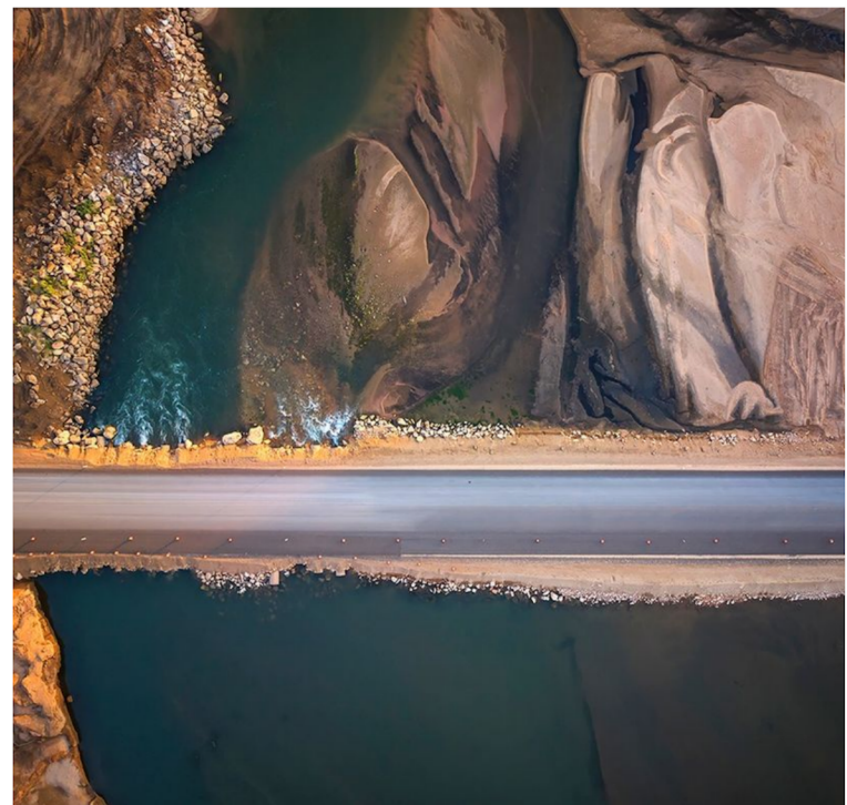
Above: Aerial view of the two-lane low level crossing.
