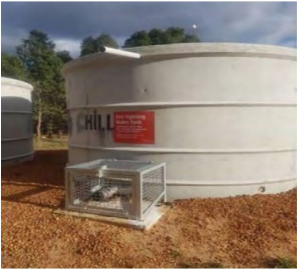
Strategic 47,000 Litre Concrete Tank & Protected Fittings
