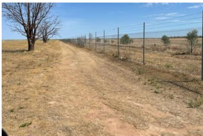
Aerodrome perimeter fence
