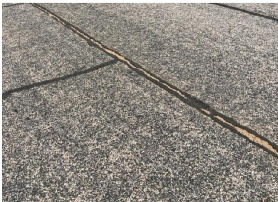
Note the sand to 'bulk out' the crack patching
