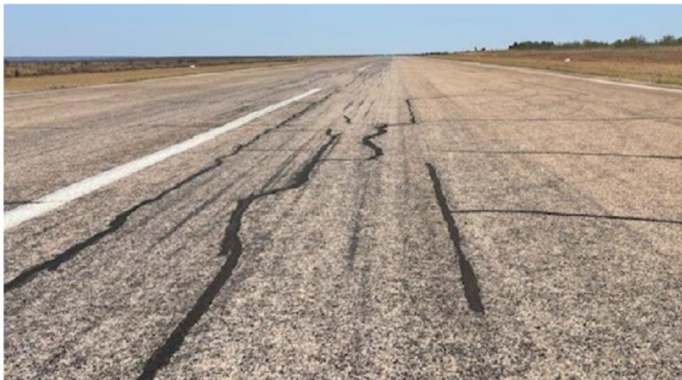
Typical crack patching.
