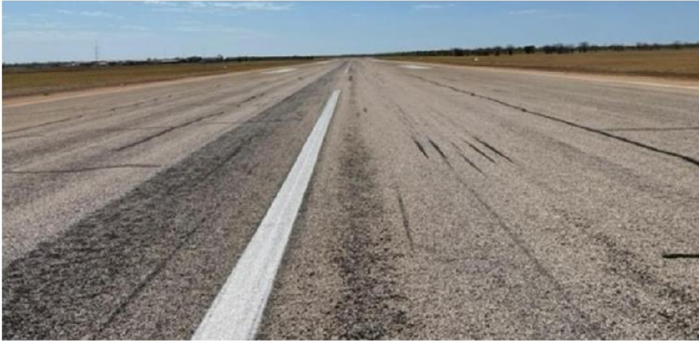
General photo West to East
