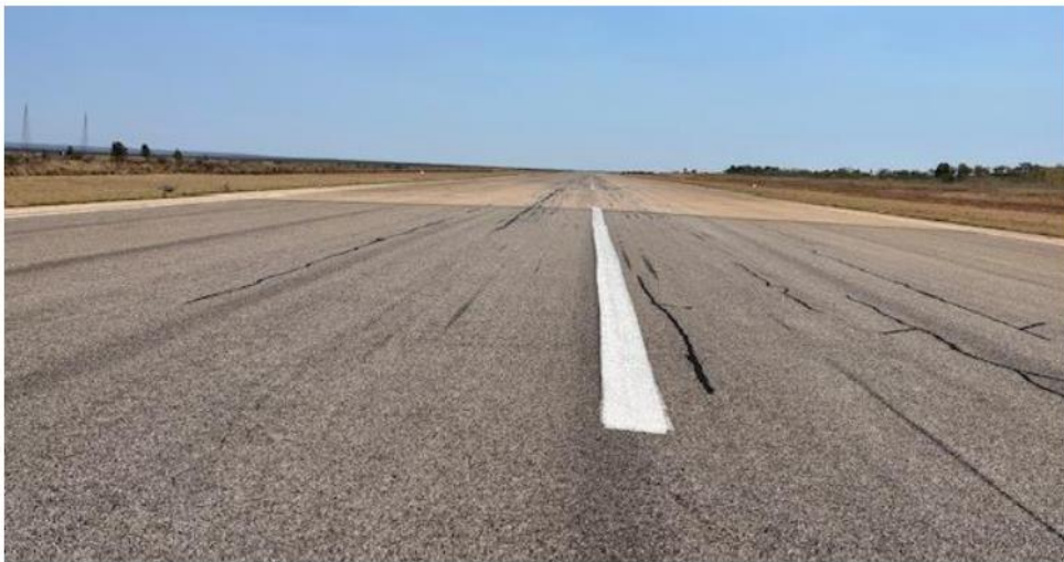
Typical view south to north
