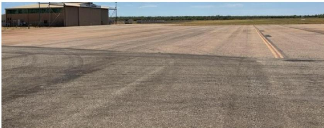
Apron showing varying seal types
