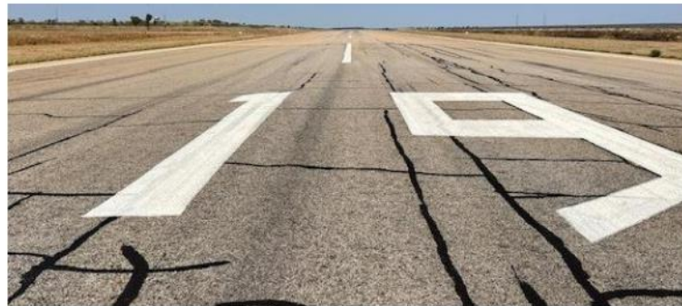
Runway 19 Line Markings
