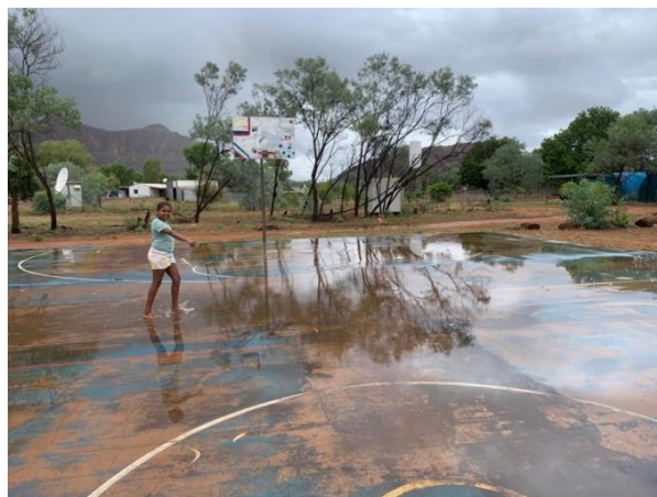
Figure 6 - The existing court in rainy days
