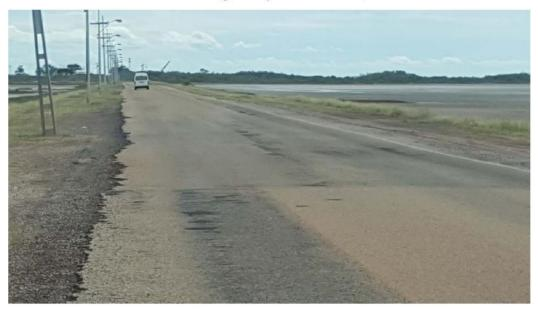
Edge Break, Jetty Rd - Condition 4, Poor
