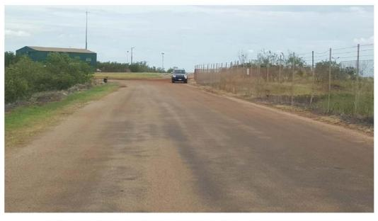
Flushing (bleeding), Jetty Boat Ramp Access Road - Condition 5, Very Poor
