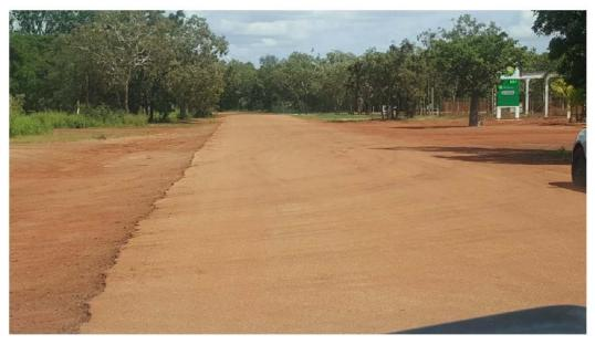
Edge Drop Off, Rodgers St – Condition 4, Poor
