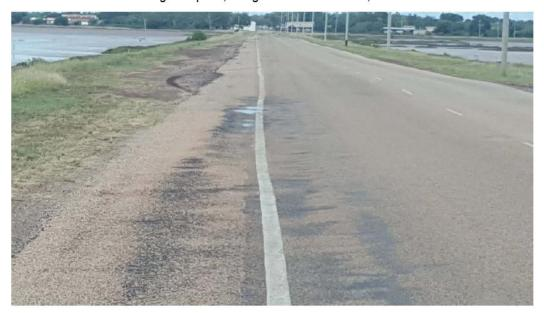
Deformation (rutting), Jetty Rd - Condition 4, Poor
