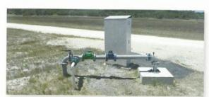
Water meter installed on galvanised headworks. Direction of flow is R to L.
