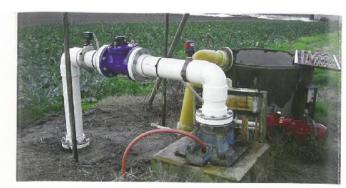
A correctly installed meter, it has no off-takes before the meter, and the required amount of pipe either side of the meter.
