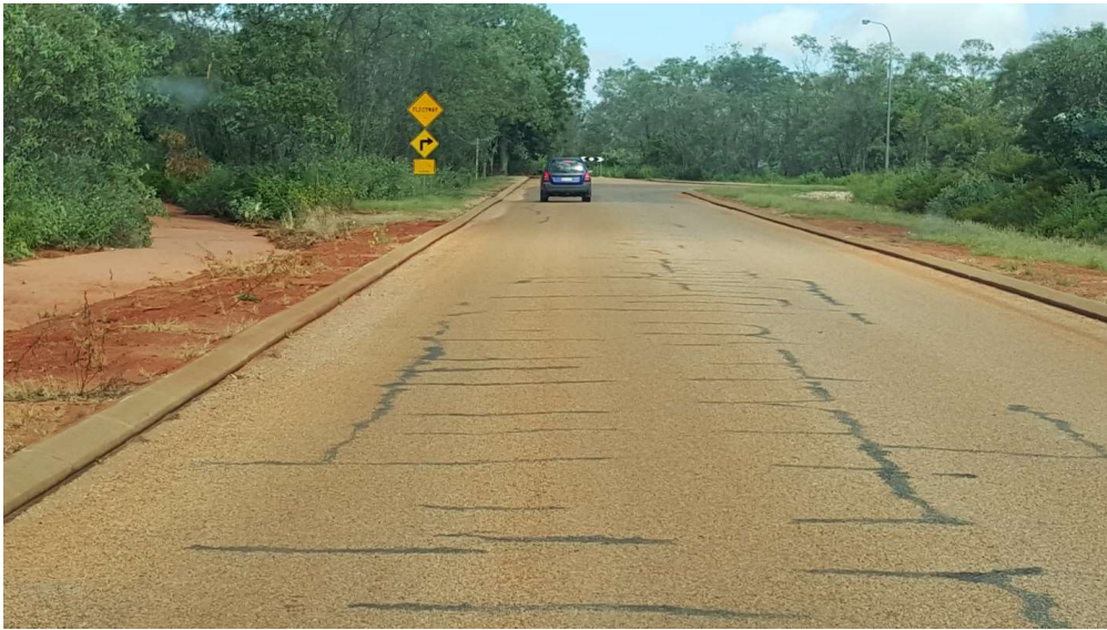
Block Cracking, Fitzroy St – Condition 3, Fair
