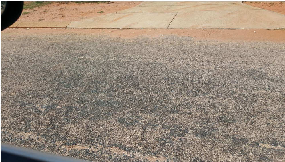
Polishing, Short St – Condition 5, Very Poor
