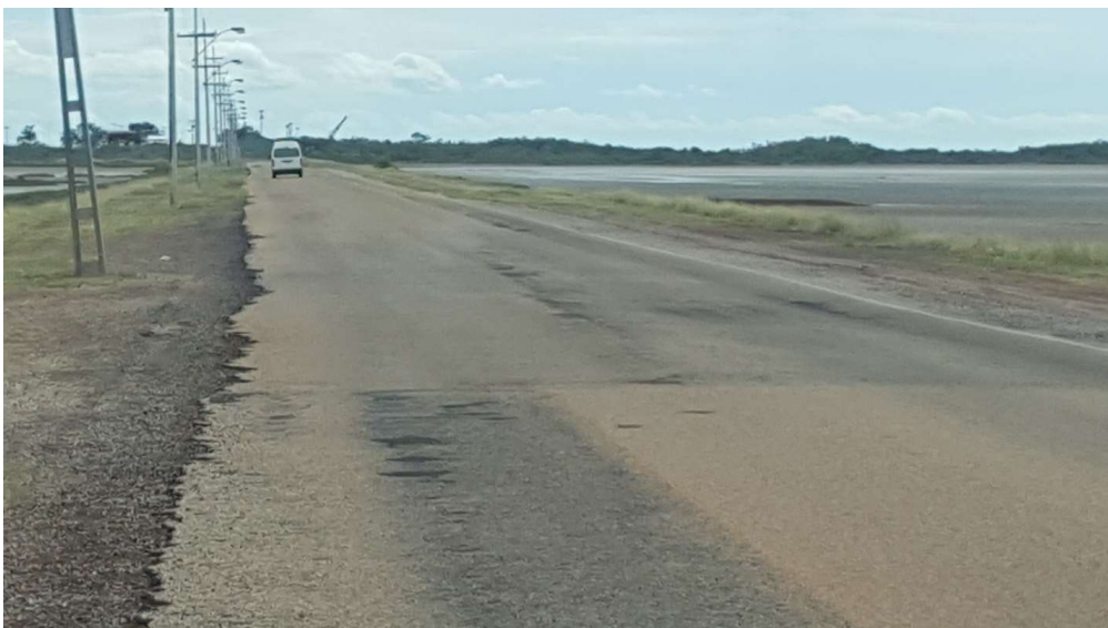
Edge Break, Jetty Rd – Condition 4, Poor
