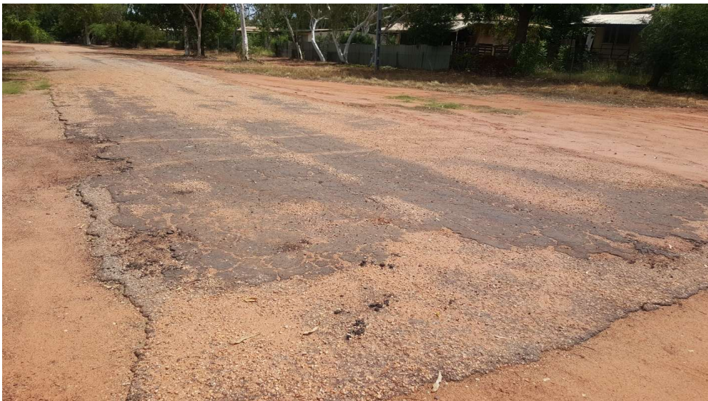
Stripping, Rowell Crt – Condition 5, Very Poor
