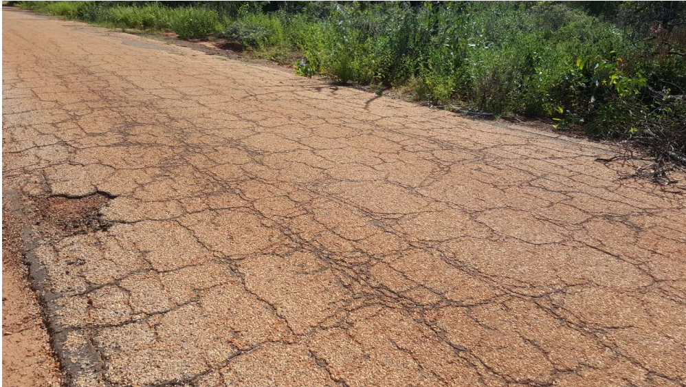
Crocodile Cracking, Granville St – Condition 5, Very Poor
