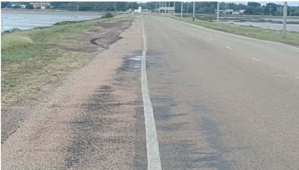
Deformation (rutting), Jetty Rd – Condition 4, Poor
