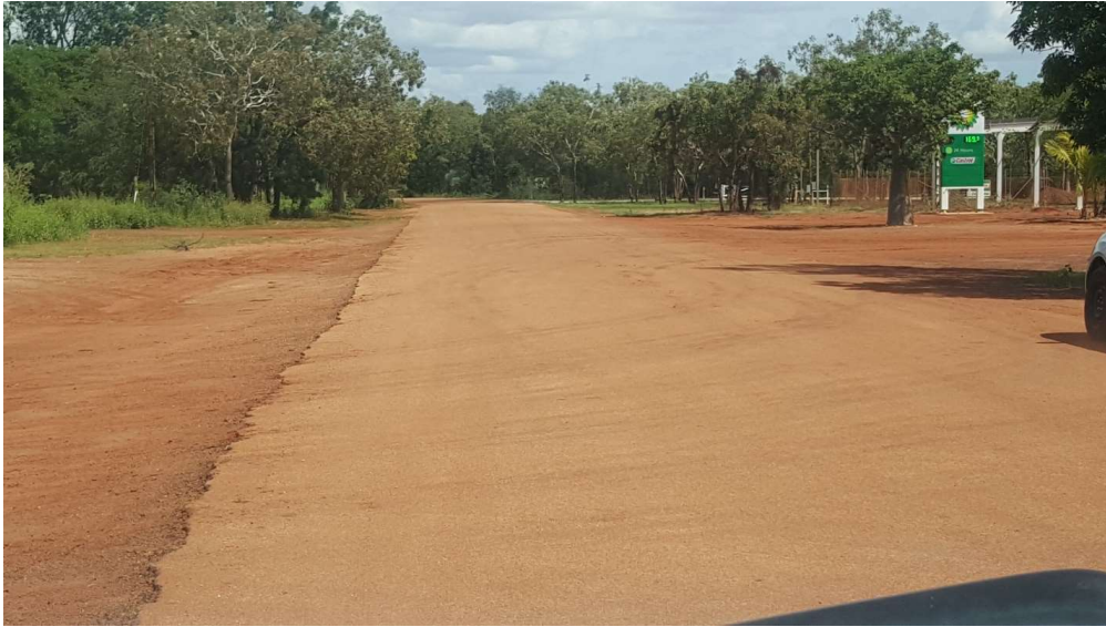
Edge Drop Off, Rodgers St – Condition 4, Poor
