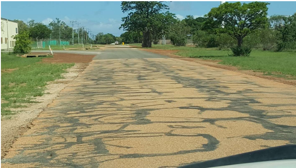
Transverse Cracking, Wodehouse St – Condition 5, Very Poor
