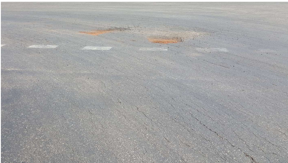
Deformation (shoving), Jetty Access Road – Condition 4, Poor
