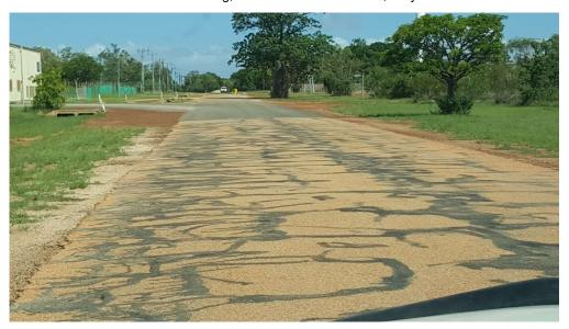
Transverse Cracking, Wodehouse St – Condition 5, Very Poor
