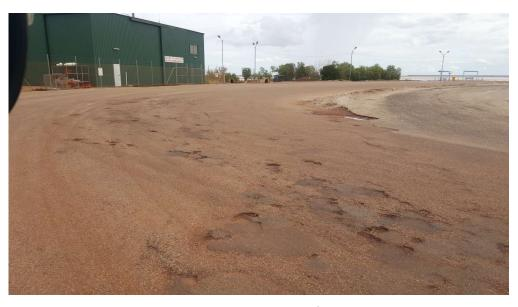
Potholing, Jetty Boat Ramp Access Road - Condition 5, Very Poor
