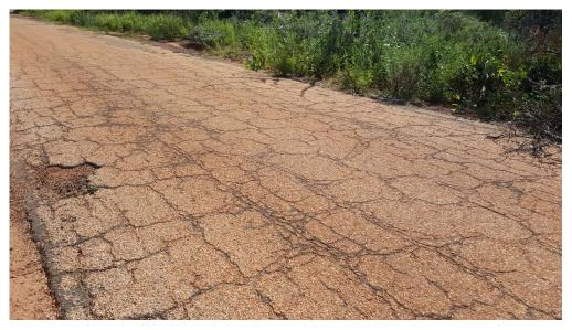
Crocodile Cracking, Granville St - Condition 5, Very Poor
