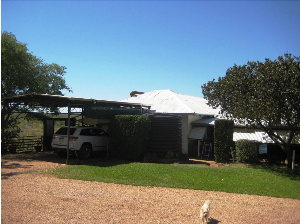
▲ P3 Northern, semi-detached end of Liveringa Homestead has timber framed walls clad with fibre cement sheet. The roof of this area may or may not be replaced subject to budget constraints. (JTA 27 April 2016)
