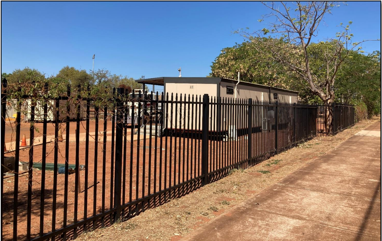
Two (2) prefabricated transportable buildings – south east corner of Subject land
