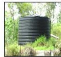
Old or unsealed rainwater tanks
