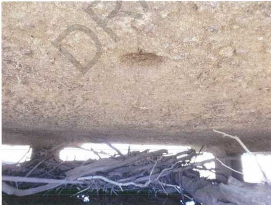
Photo No. 32: LHS span 34, top deck slab soffit. (Taken: 20-Jun-2016)
