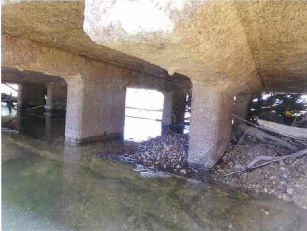
Photo No. 41: RHS at pier 30. (Taken: 20-Jun-2016)
