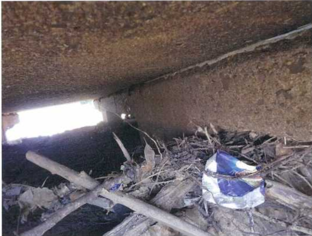
Photo No. 19: LHS span 9, top deck A2 end. (Taken: 20-Jun-2016)
