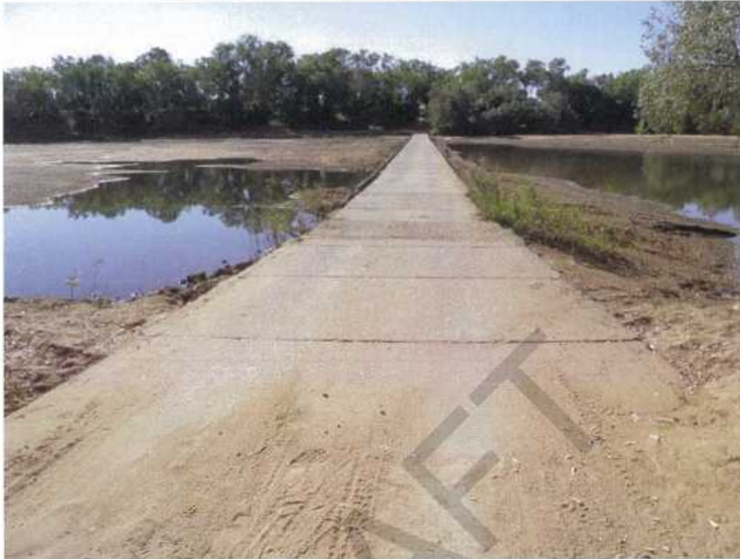
Photo No. 5: A2 end view (Taken: 20-Jun-2016)
