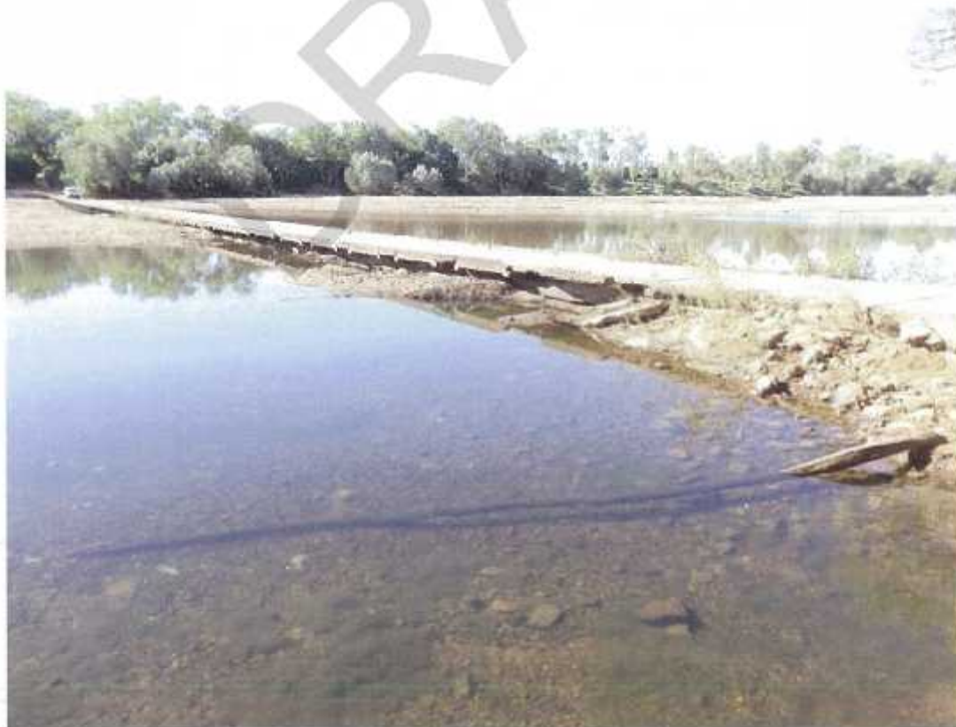
Photo No. 52: RHS elevation from abutment 2 end. (Taken: 20-Jun-2016)
