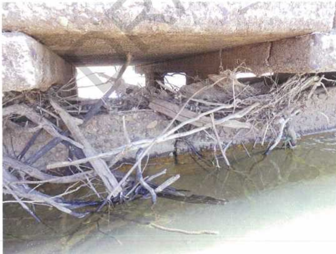
Photo No. 24: LHS pier 20. (Taken: 20-Jun-2016)
