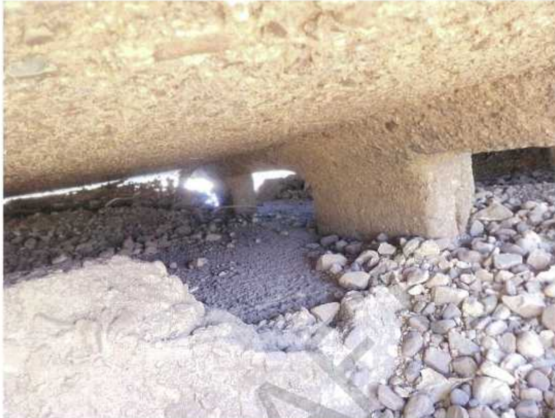
Photo No. 35: LHS span 44. (Taken: 20-Jun-2016)
