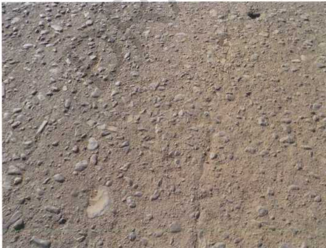
Photo No. 12: Minor cracking to the deck surface - Spans 24 and 25 (Taken: 20-Jun-2016)
