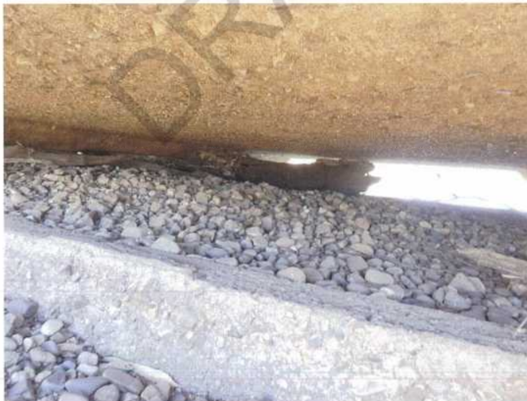
Photo No. 34: LHS span 42. (Taken: 20-Jun-2016)
