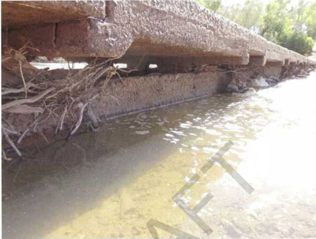
Photo No. 23: LHS span 20. (Taken: 20-Jun-2016)
