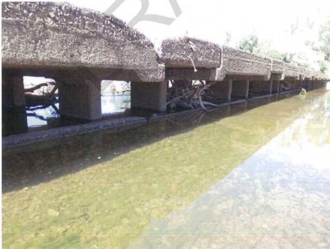
Photo No. 42: RHS at span 24 to span 28. (Taken: 20-Jun-2016)
