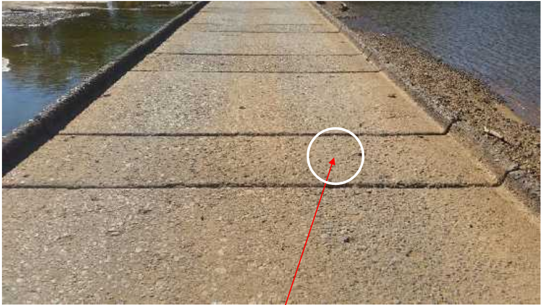
104058 – Diagonal crack
