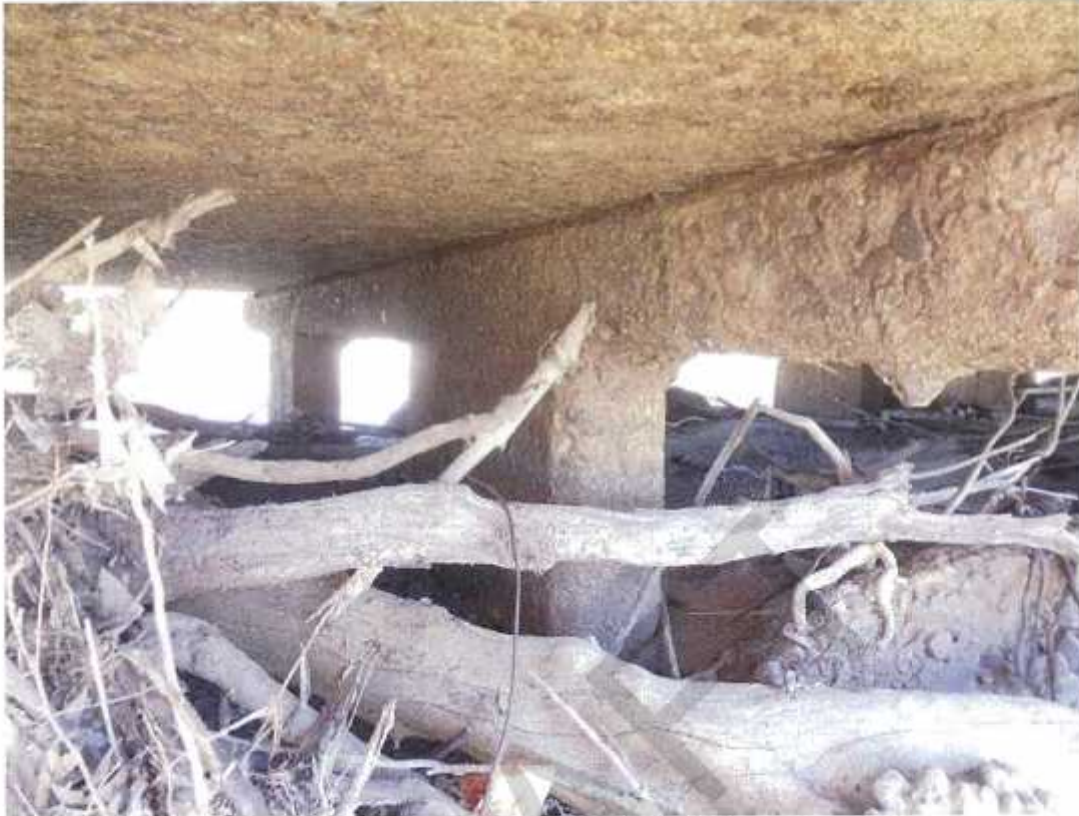
Photo No. 25: LHS at pier 21, legs to top deck. (Taken: 20-Jun-2016)
