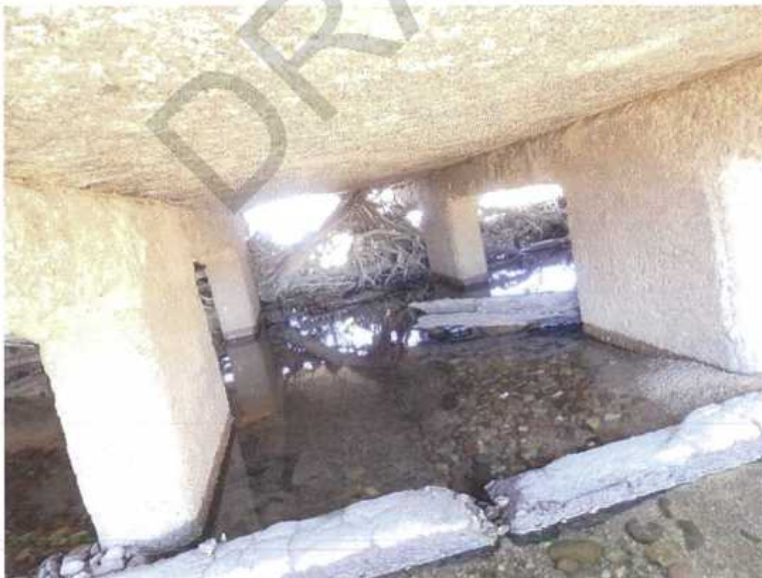
Photo No. 40: RHS at pier 36. (Taken: 20-Jun-2016)
