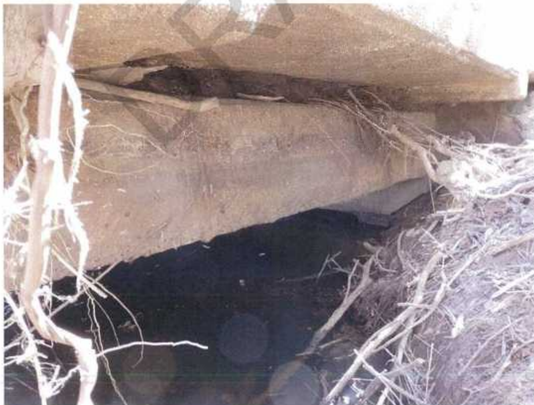
Photo No. 16: LHS span 5. (Taken: 20-Jun-2016)
