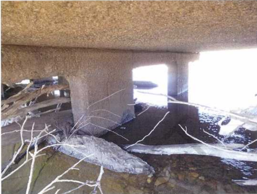
Photo No. 27: LHS at pier 22, top deck legs. (Taken: 20-Jun-2016)
