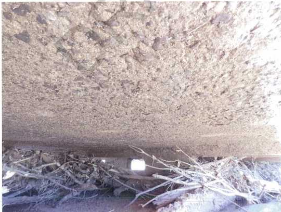
Photo No. 26: LHS span 22, top deck soffit. (Taken: 20-Jun-2016)
