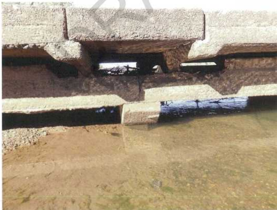
Photo No. 44: RHS at pier 9. (Taken: 20-Jun-2016)
