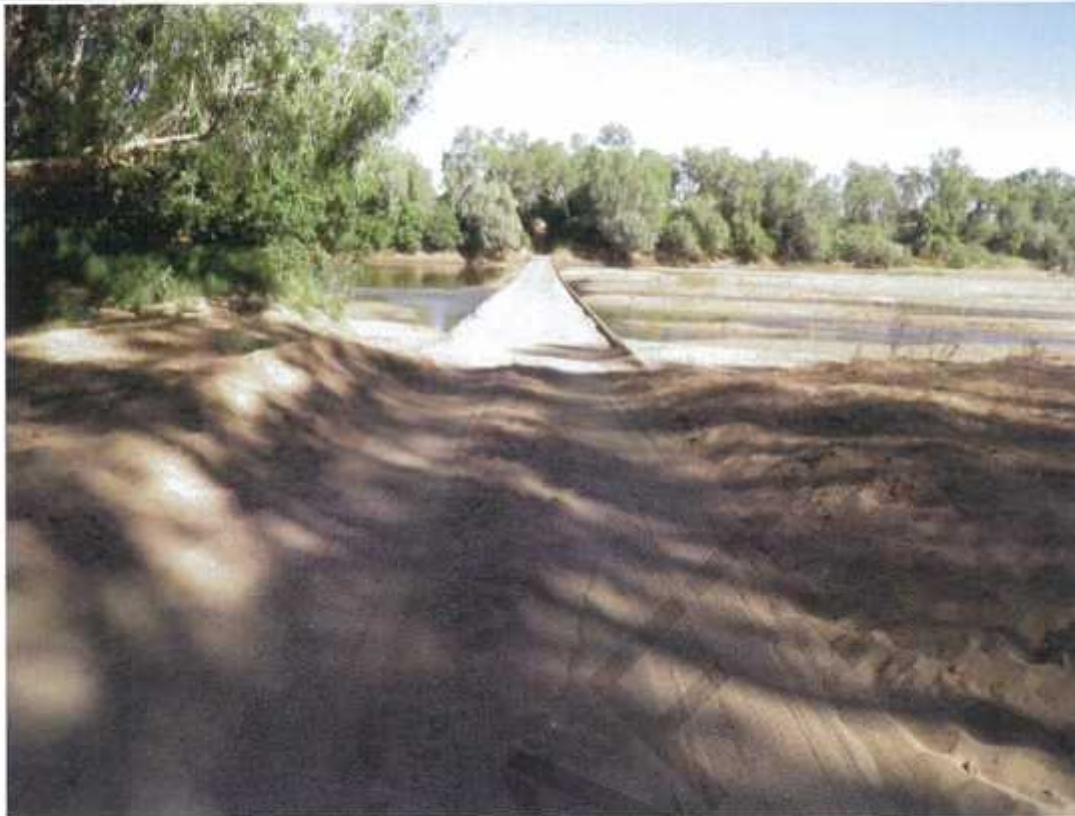
Photo No. 1: A1 end view (Taken: 20-Jun-2016)
