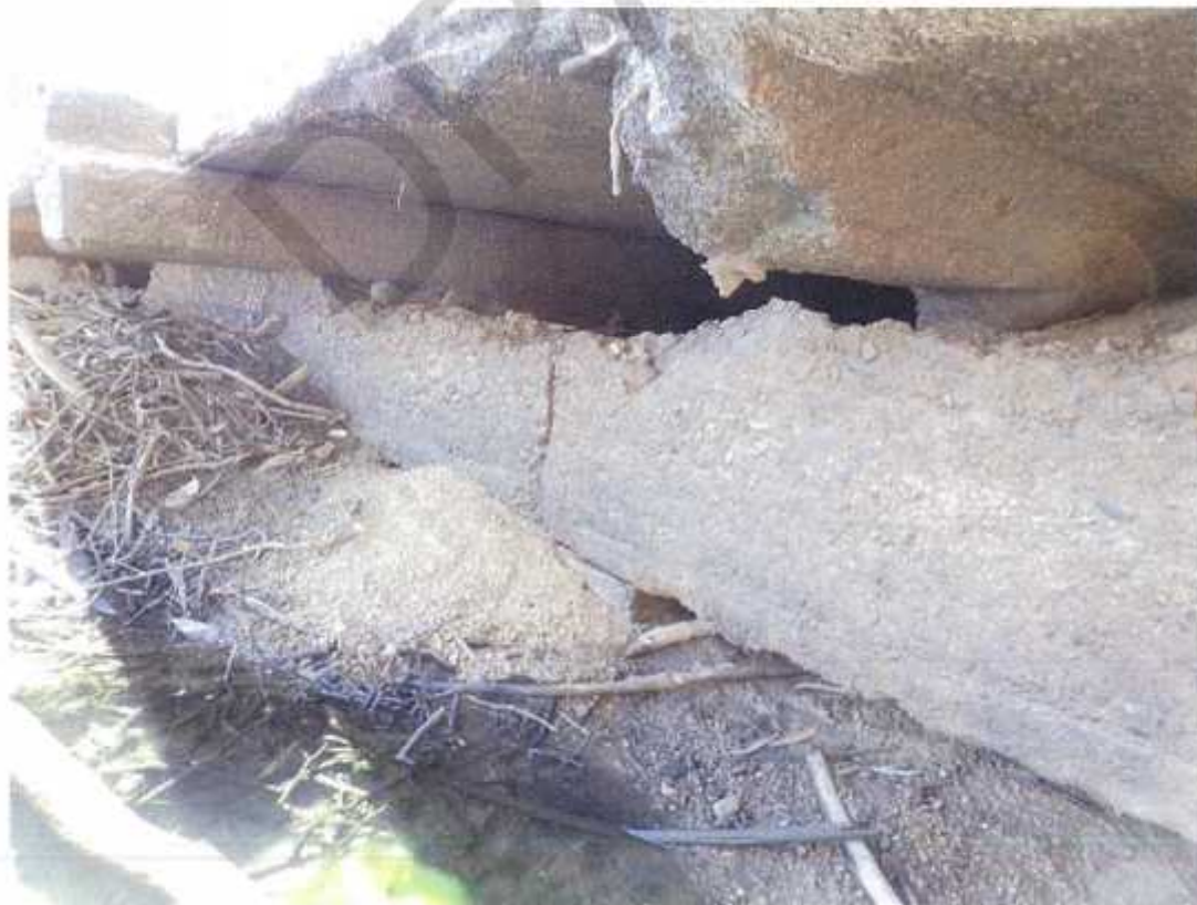
Photo No. 38: RHS at pier 47. (Taken: 20-Jun-2016)
