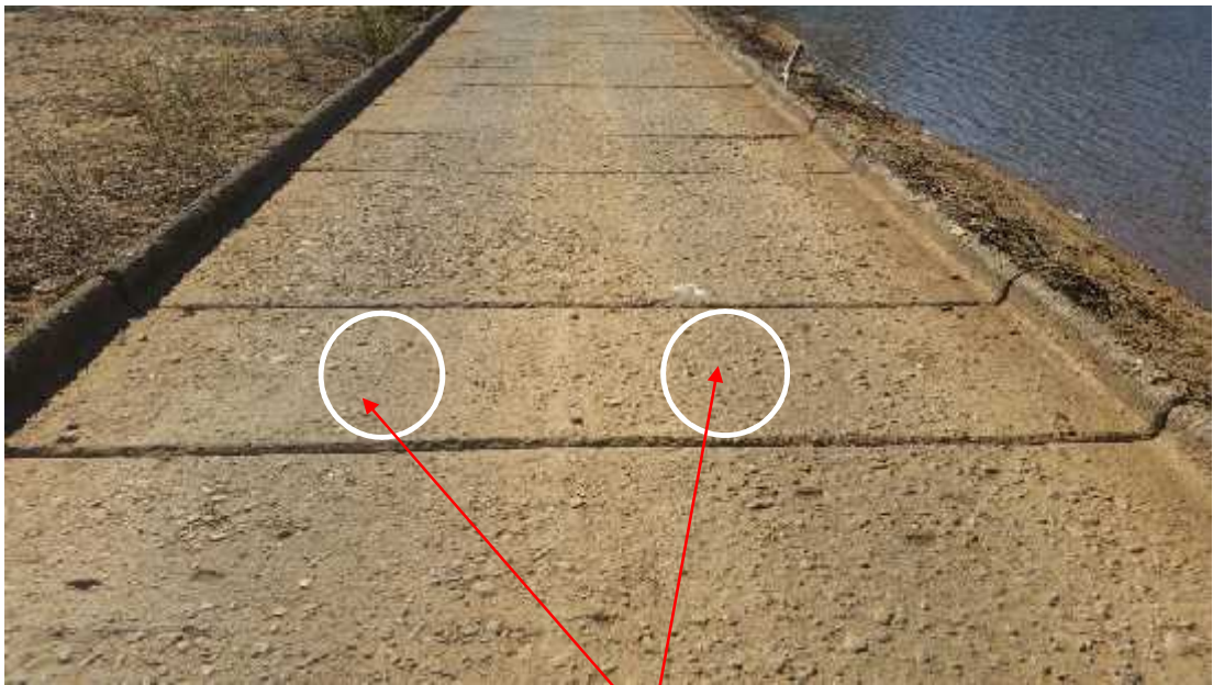
140005 – Longitudinal cracks
