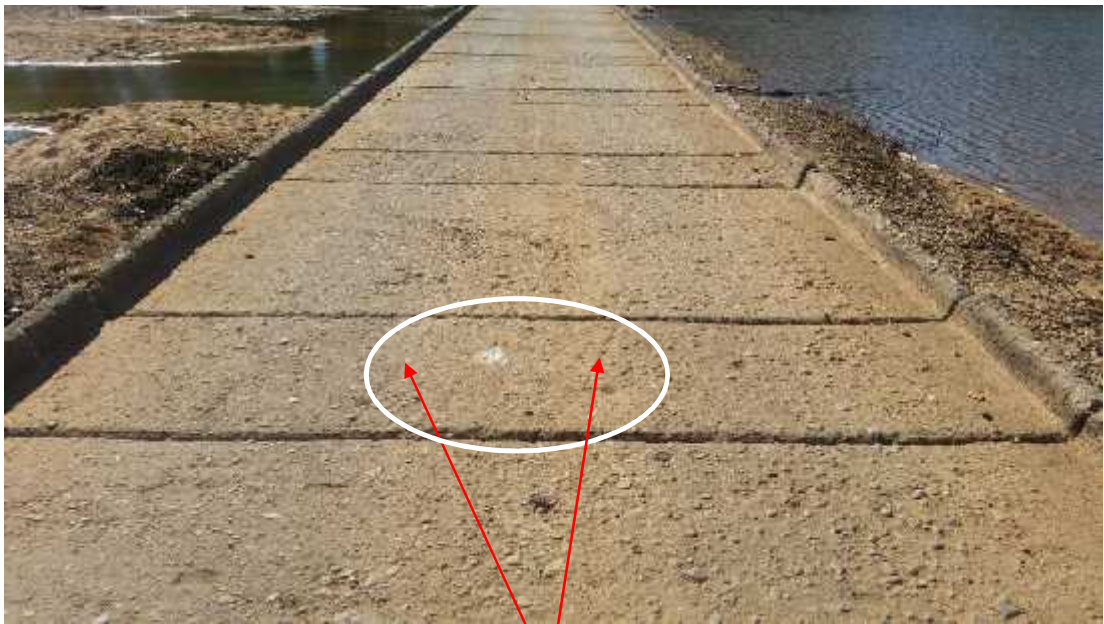
140030 – Longitudinal cracks
