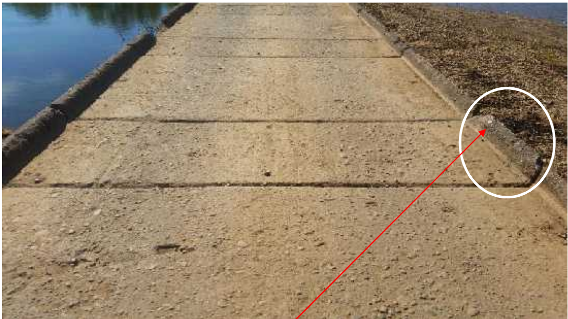
135911 – Kerb spalled
