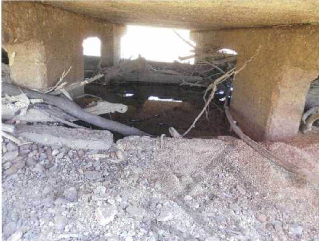
Photo No. 33: LHS at pier 39, legs for main deck. (Taken: 20-Jun-2016)
