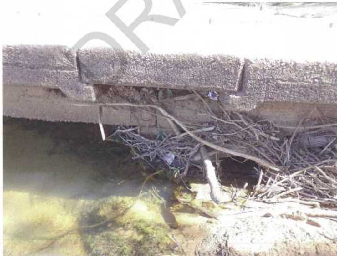
Photo No. 22: LHS pier 9 link top slab. (Taken: 20-Jun-2016)
