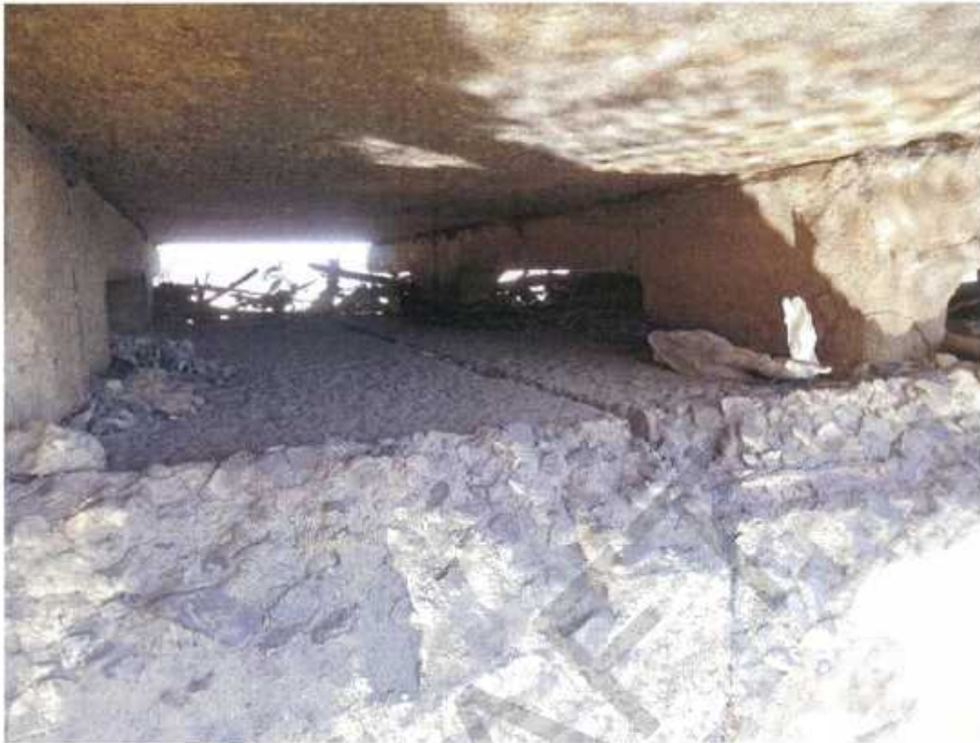
Photo No. 45: RHS at pier 9. (Taken: 20-Jun-2016)
