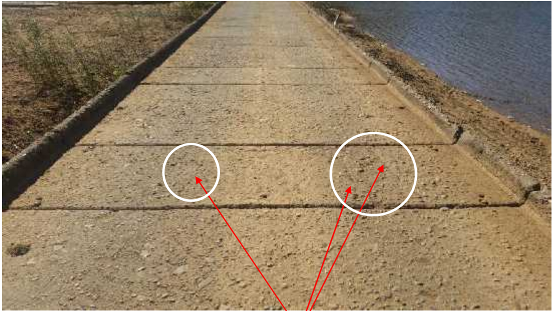
140000 – Longitudinal cracks
