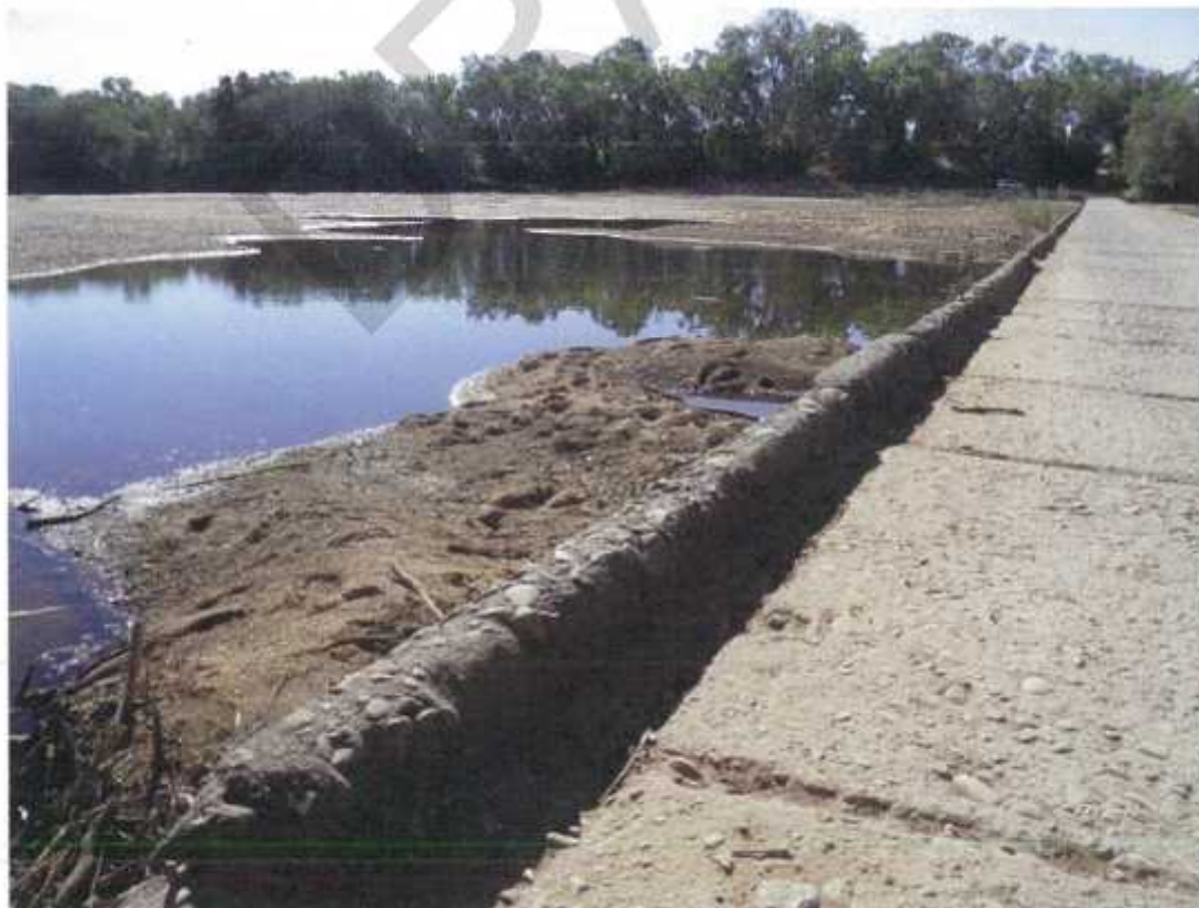
Photo No. 4: RHS (Taken: 20-Jun-2016)
