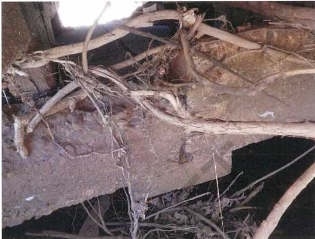
Photo No. 15: LHS pier 5. (Taken: 20-Jun-2016)
