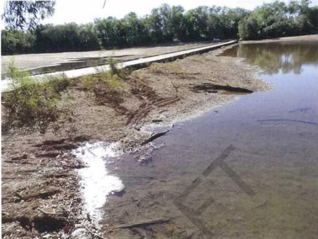
Photo No. 51: LHS elevation from abutment 2 end. (Taken: 20-Jun-2016)
