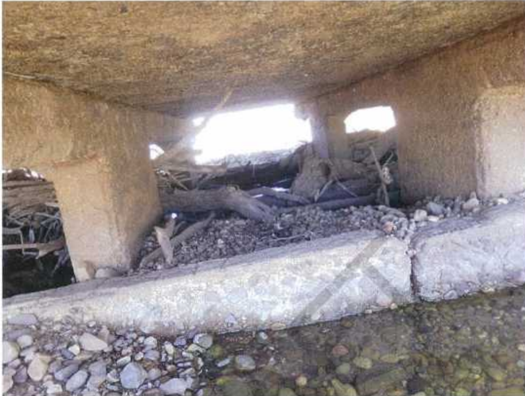
Photo No. 39: RHS at pier 39. (Taken: 20-Jun-2016)
