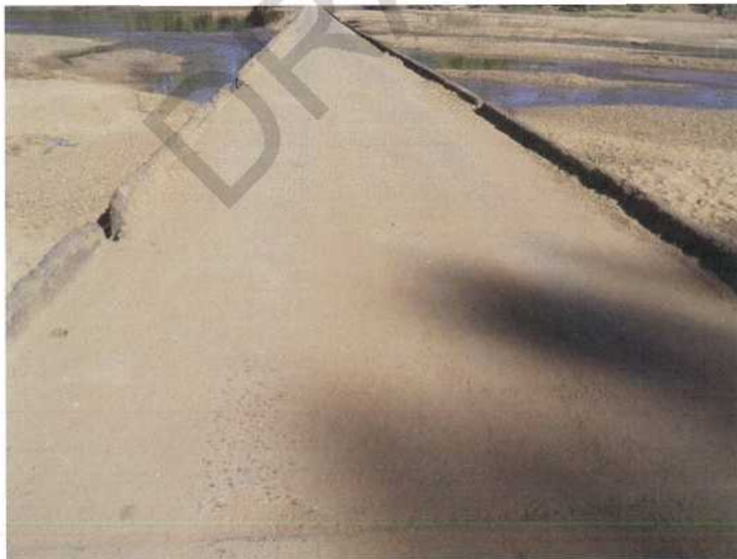
Photo No. 2: Deck (Taken: 20-Jun-2016)
