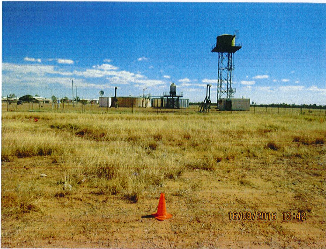
View from proposed facility looking west
