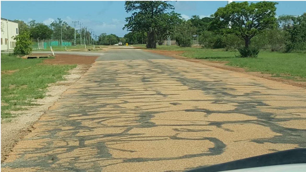
Transverse Cracking, Wodehouse St – Condition 5, Very Poor
