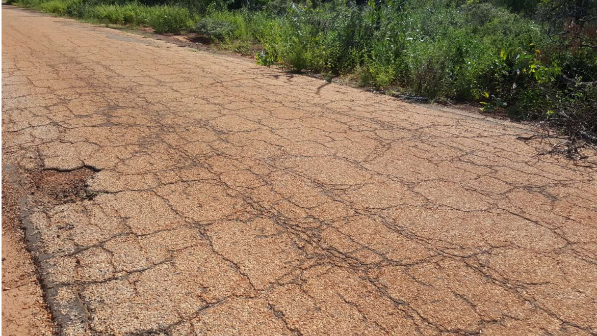
Crocodile Cracking, Granville St – Condition 5, Very Poor
