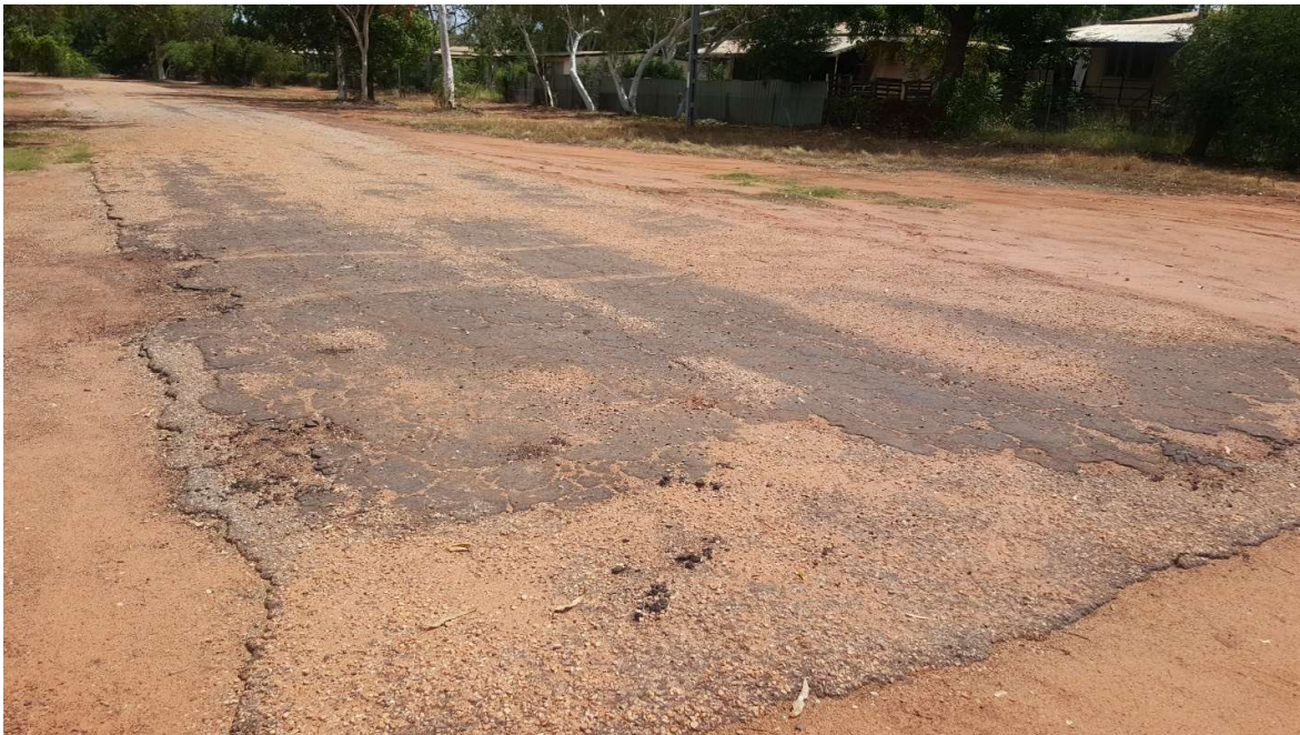
Stripping, Rowell Crt – Condition 5, Very Poor
