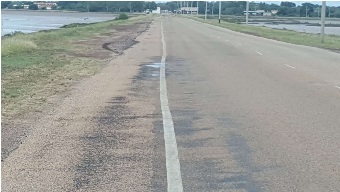
Deformation (rutting), Jetty Rd – Condition 4, Poor
