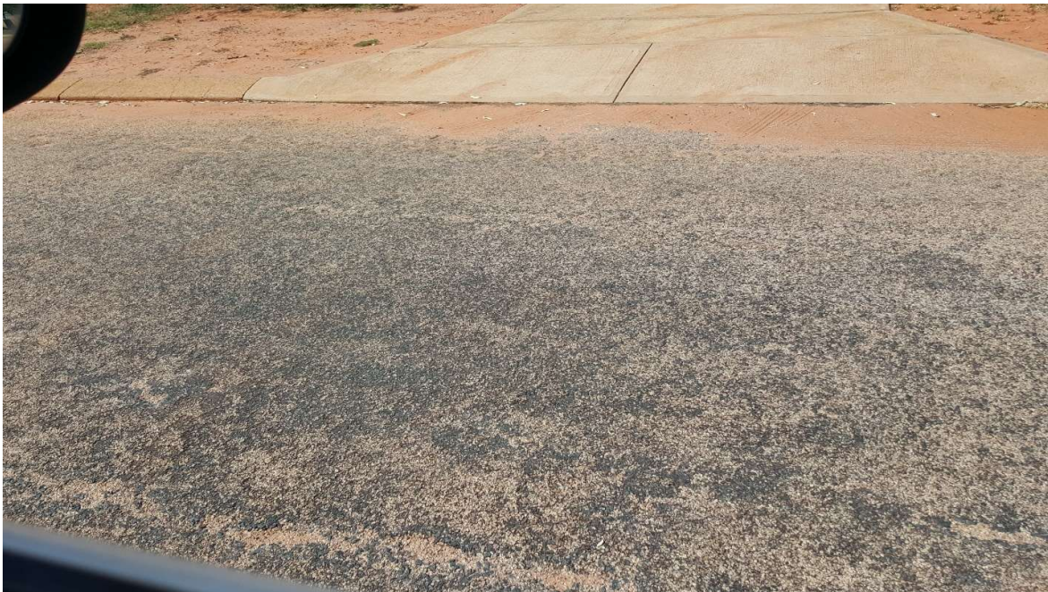
Polishing, Short St – Condition 5, Very Poor
