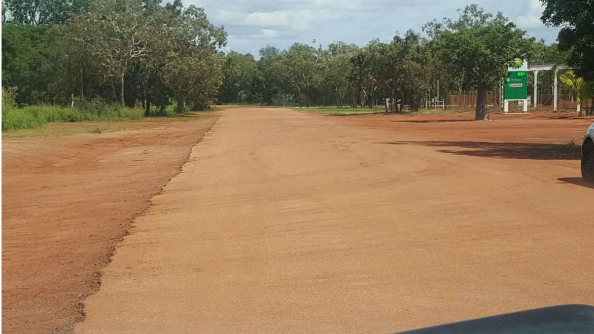
Edge Drop Off, Rodgers St – Condition 4, Poor
