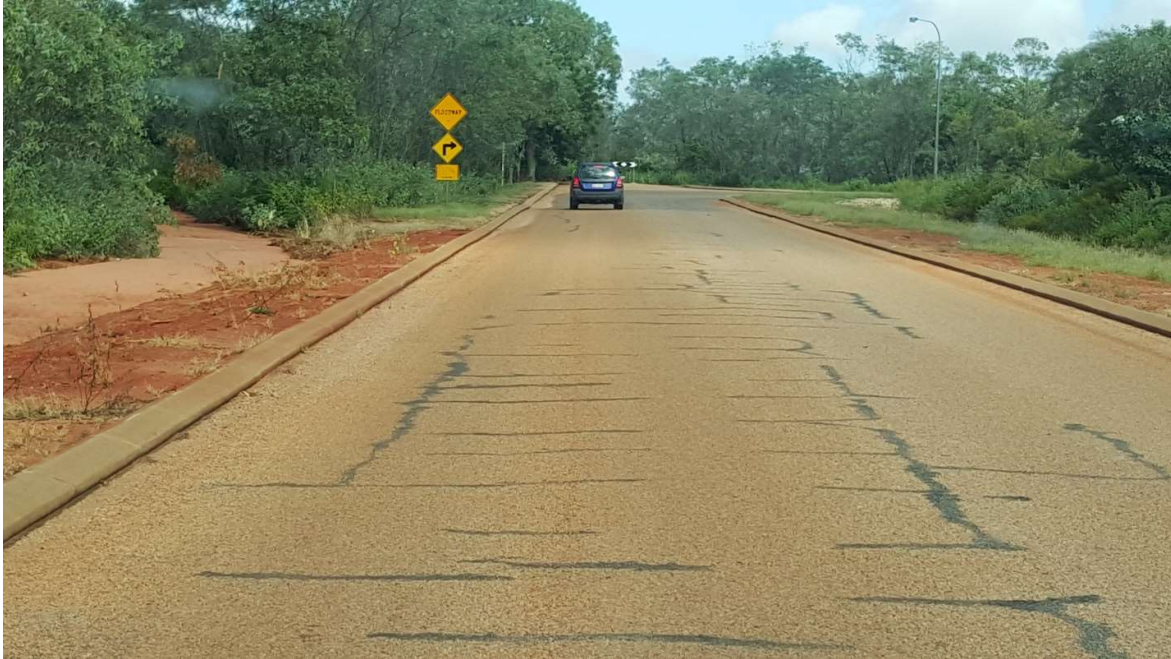
Block Cracking, Fitzroy St – Condition 3, Fair
