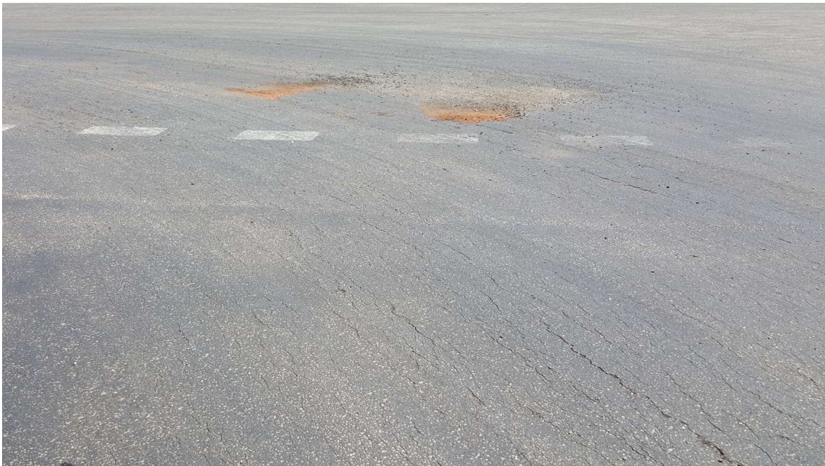
Deformation (shoving), Jetty Access Road – Condition 4, Poor
