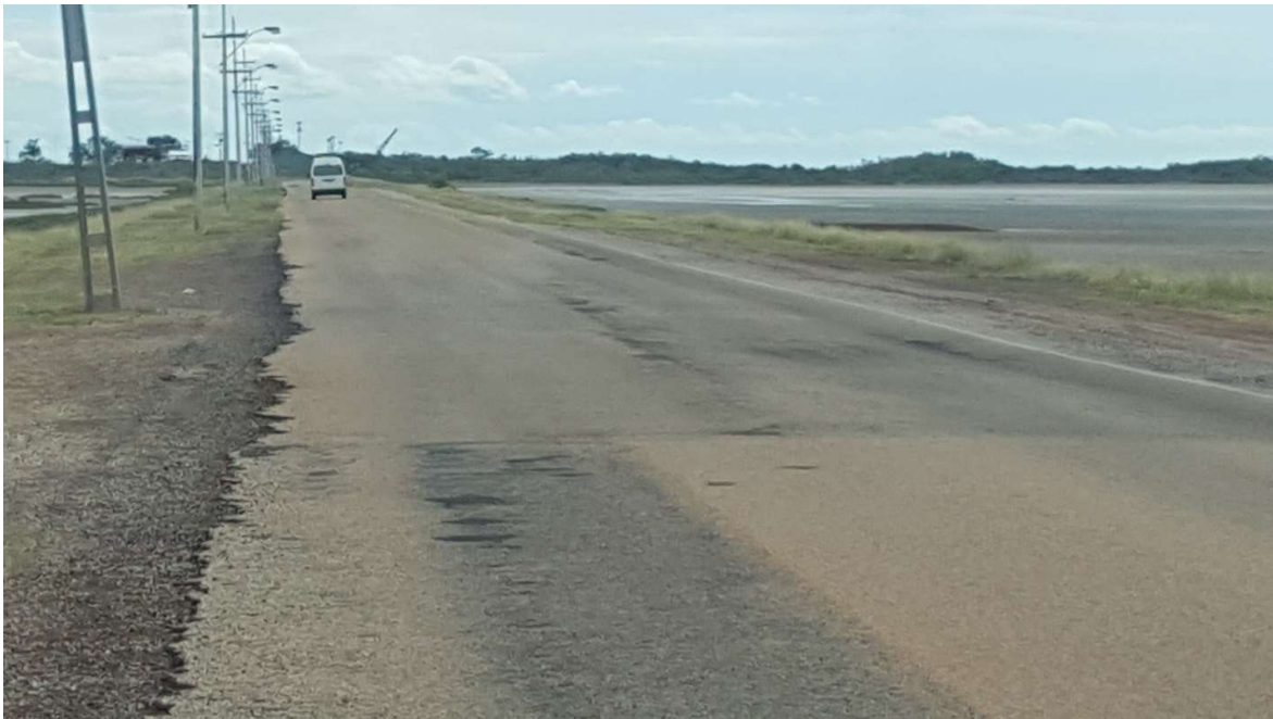
Edge Break, Jetty Rd – Condition 4, Poor
